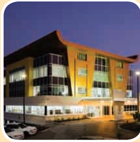
New Administration Building
